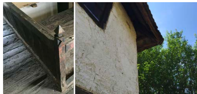
Figure 17: Left - Detail of fence on gallery; Right - Finishing of exterior wall surfaces: white painted clay mortar with straw and chaff
