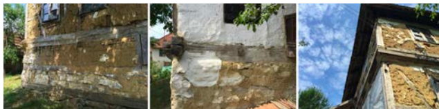
Figure 18: Details of the structural assembly of the house; Left and center - Basement wall of semi-finished stone; Right - Bondruk system with adobe fill (ground floor and first floor)
