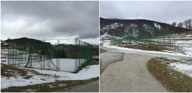
Figure 10: Bobovica village - newly built structures
