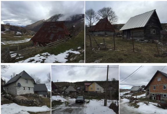
Figure 7: Bobovica village - new houses built on the walls of (demolished) traditional houses
