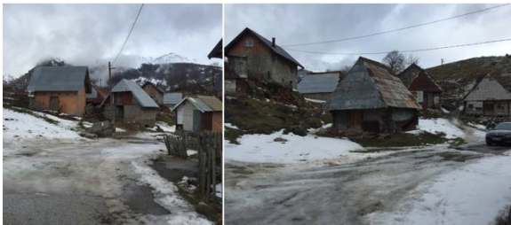
Figure 6: The Bobovica village - restored old structures of buildings
