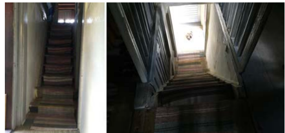
Figure 10: Ground floor-first floor staircase
